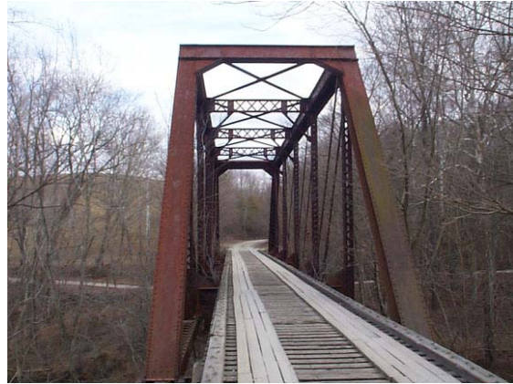
Bridge on Chesapeake & Ohio line, Carter County
