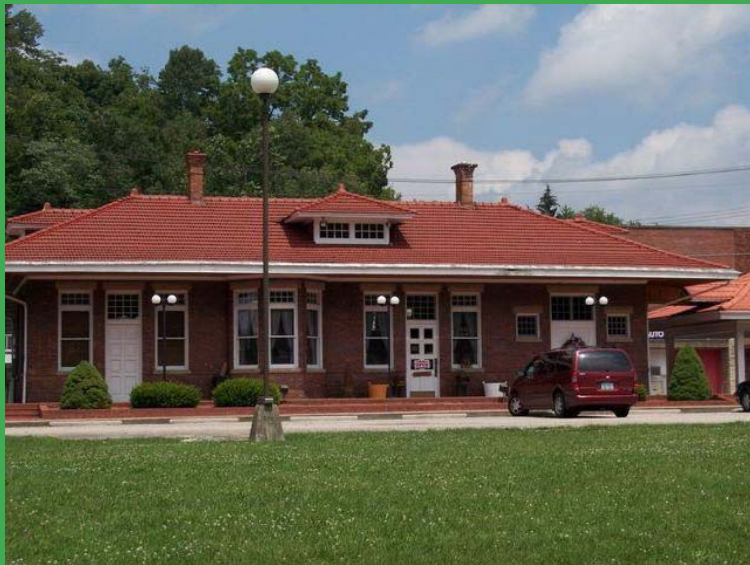
C & O Railway Depot at Olive Hill
