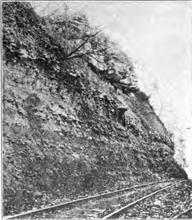
Plate 21. Deep cut on Kiniconick Branch, Chesapeake & Ohio R. R., four miles west of Carter, Carter County. Looking west. Morris Mountain member of the Logan formation, 40 feet thick, overlain by Ste. Genevieve limestone.
