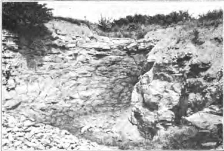
Plate 36. Quarry in Warsaw limestone at Glasgow, Ky. About 50 feet of coarse, crinoidal limestone. Looking north. This is a good exhibition of the limestone facies of the Warsaw. The rock here has the same aspect as the Warsaw has southward into Overton County, Tenn., and northward to Harrodsburg, Ind., the type locality of the "Harrodsburg" limestone, which is the partial equivalent of the Warsaw. (See Plate 39).
