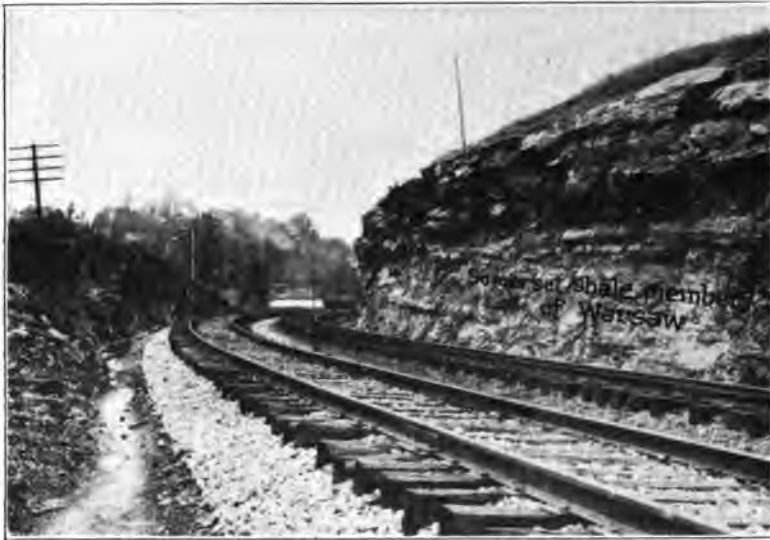
Plate 47. Cut about one-fourth mile north of railroad station at Somerset, showing Somerset shale member of the Warsaw. Layers of St. Louis limestone at top. Looking north.
