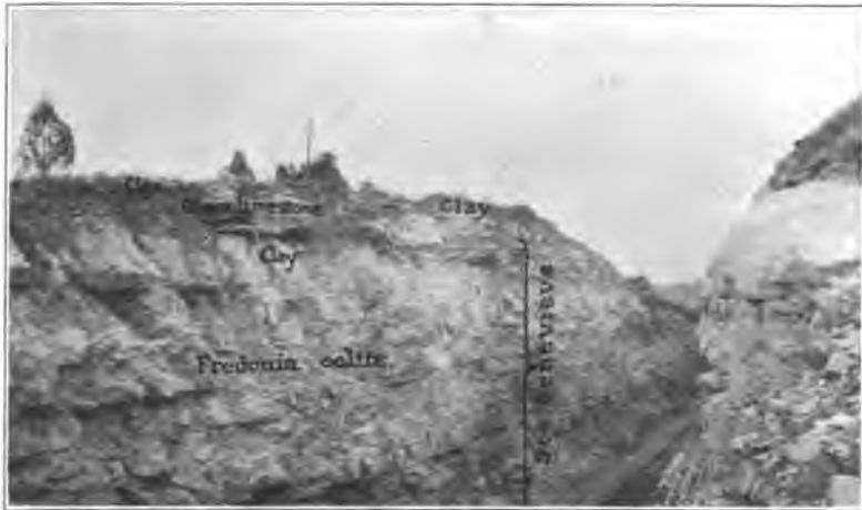
Plate 71. Cut on Cincinnati Southern Railroad one-fourth mile south of Cedar Grove and four miles south of Somerset, Ky. Looking south. Shows near top an upper layer weathering to clay, a lower layer weathering to clay, and a layer of oolite between. Beds below the lower clay are St. Genevieve (Fredonia oolite member) with Platycrinus penicillus (huntsvillae) to the top. One-half mile north the oolite bed between the two clay layers is crowded with small specimens of Pentremites principonensis ; and Mesoblastus glaber are common and one or more species of Talarocrinus are present but not common. Invariable succession from Fredonia oolite to Gasper oolite along Cumberland escarpment. See Plates 70 to 73 inclusive.
