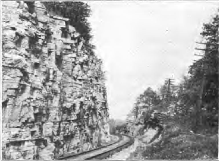
Plate 37. "Harrodsburg facies" of the Warsaw limestone extending up to the Somerset shale member shown in Plate 49. Cut on the Louisville & Nashville Railroad one-half to one mile north of the tunnel at Tunnel Hill. Looking north. The shaly layer shown in Plate 43 appears at base of cut at the farther end.
