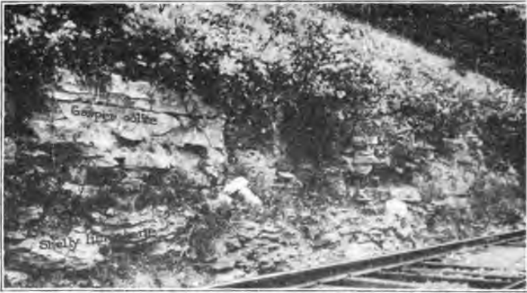
Plate 73. Cut on Louisville & Nashville R. R. on Kentucky River about 2 miles west of Heidelberg. At bottom, argillaceous, gray, shelly limestone at base of Gasper oolite. Looking east.
