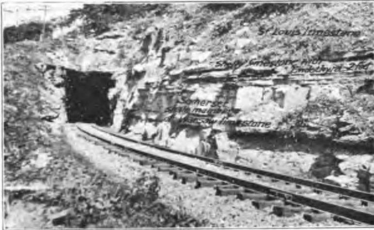
Plate 48. South portal of tunnel on Illinois Central Railroad about four miles north of Muldraugh, Ky. Cut in Somerset shale member of the Warsaw. Looking north.
