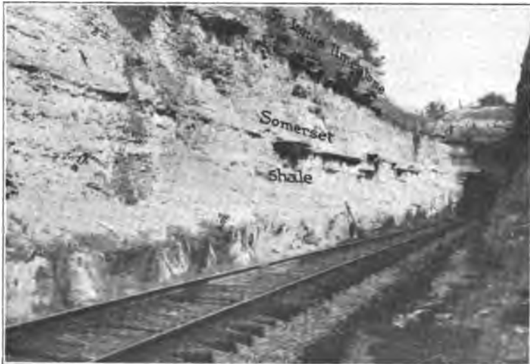
Plate 49. Cut at south end of tunnel on the L. & N. R. R. at Tunnel Hill, about four miles north of Elizabethtown, Hardin County. Cut in the Somerset shale member of the Warsaw formation. Looking northwest. This is the highly fossiliferous bed yielding the fossils in the glades on the hill at the well-known locality about 2\frac{1}{2} miles southwest of Clesburg, Ky. The light colored bed above the portal is the base of the St. Louis limestone; the thick, dark bed just above the shale is in the Warsaw. See Plate 48.
