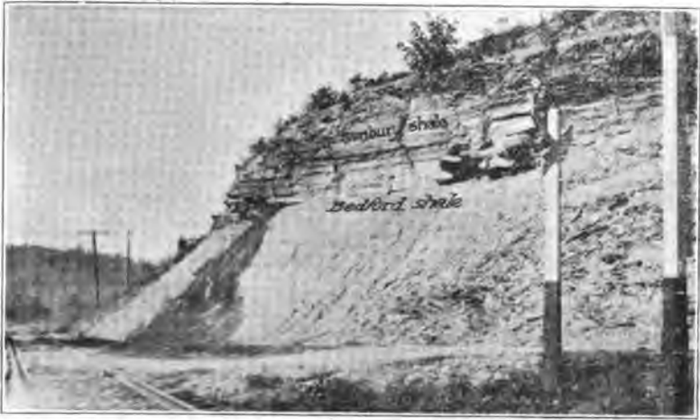
Plate 3. Sunbury shale, 16 feet thick, underlain by Bedford shale, 20 feet thick. Cut on Chesapeake & Ohio Railroad at Bluestone siding near Rockville, five miles southwest of Morehead. Looking west.
